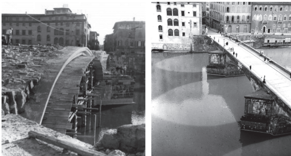
Fig. C-24. Left: The Ponte a Santa Trinita during the reconstruction of the central arch, 1956; Right: The bridge just after its completion, 1958 (Gizdulich Archive, Florence, reproduced from Belli).
