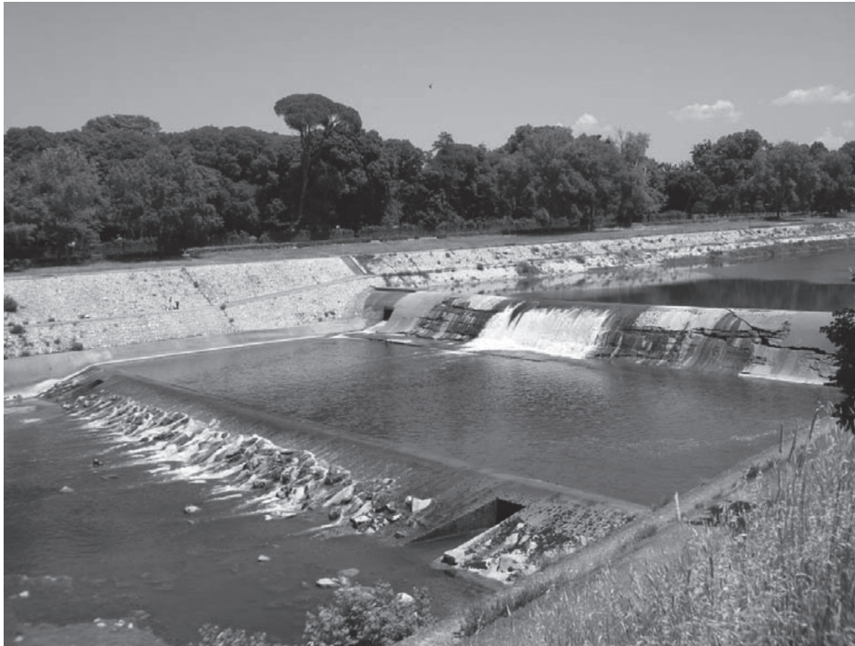
Fig. C-12. The Isolotto weir and counter-weir.
